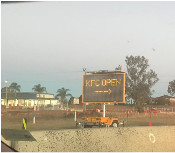
Picture taken 22 nd May 2018 from a car of a motorway construction site along the A9 in Penrith – using road signs to advertise fast food.
