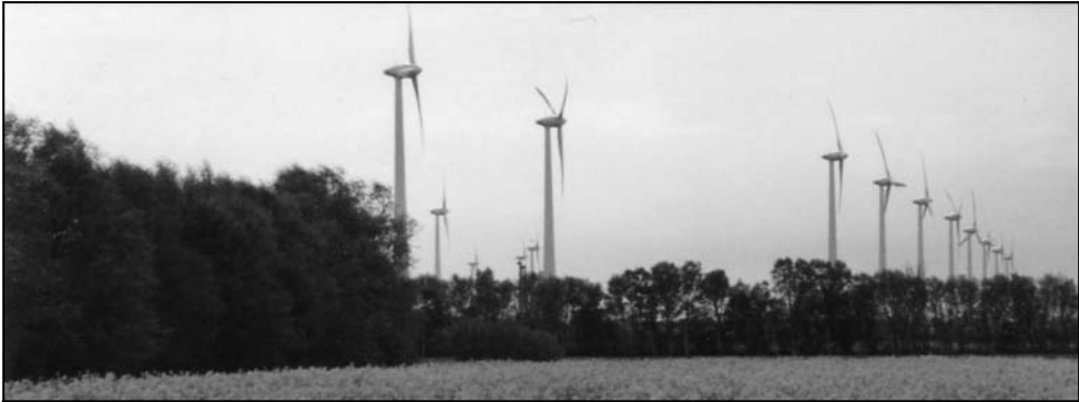
Figure IV.1: the Rhede wind farm, view from the north-northwest
