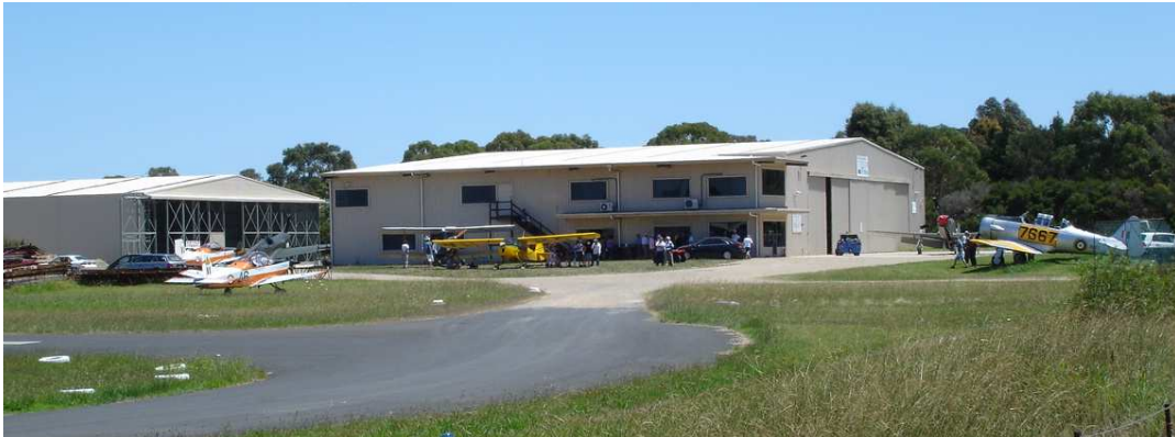
Tyabb Airfield Photograph copyright Tyabb & District Ratepayers, Business & Environment Group Inc
