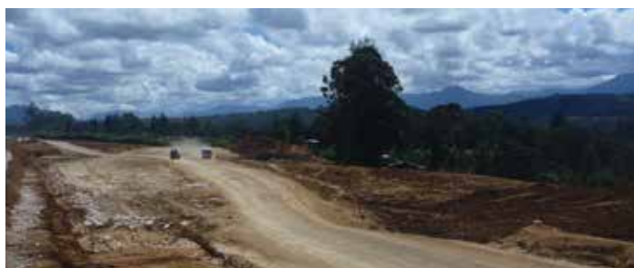
Runway extension work next to Tari Airport, 2011. Photo credit: James McIlraith/University of Otago.
