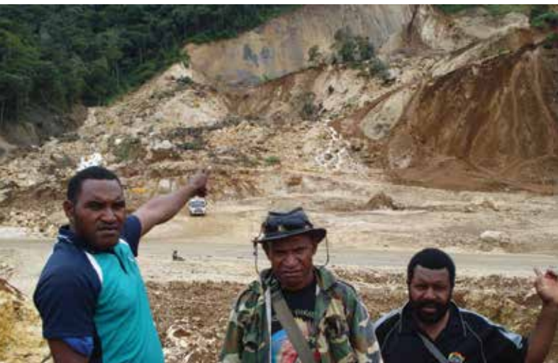
The Tumbi Landslide January 2012. Photo credit: LNGWatchPNG.blogspot.com.
