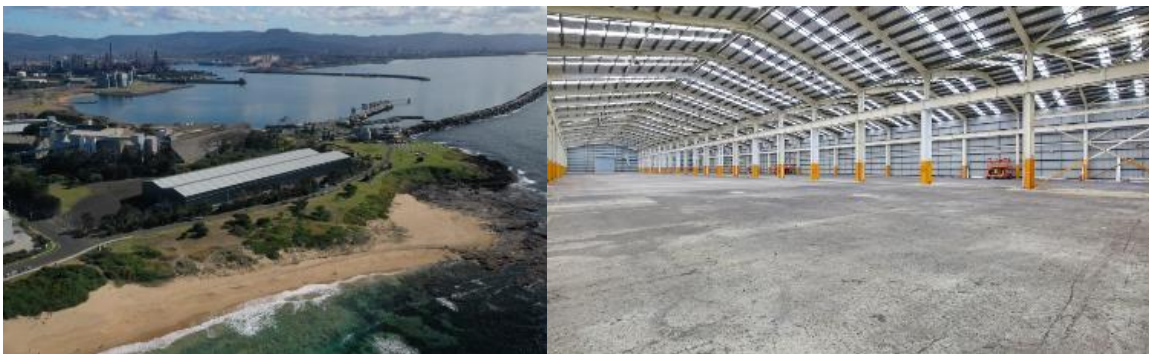
Figure 1 Hysata's new Port Kembla hydrogen electrolyser manufacturing facility
