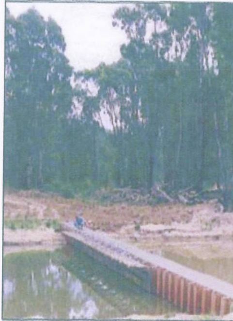
Installation of Moira Lake regulator. (Photo courtesy of David Leslie)
