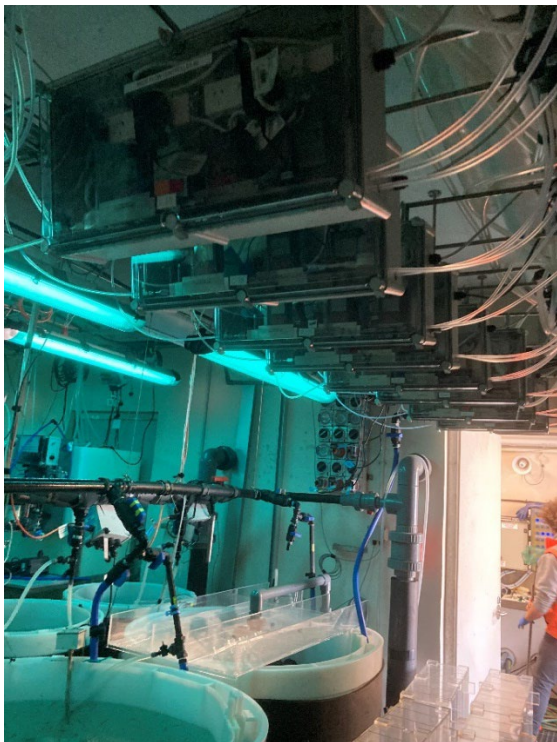
Figure 2: WHS issues – Electrical power outlets and controls located in the same wet space as livestock
