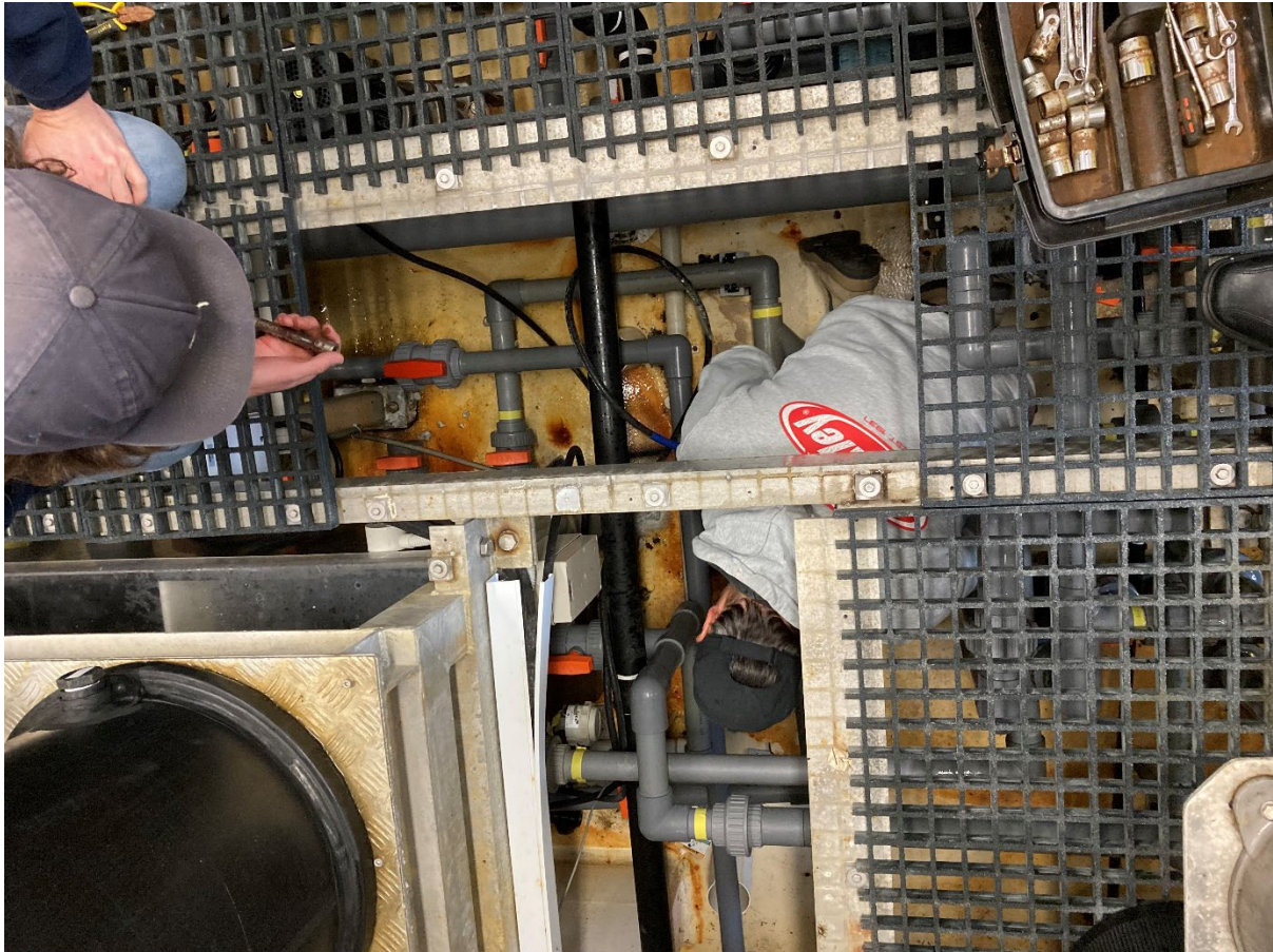
Figure 1: WHS issues - Working in a confined space
