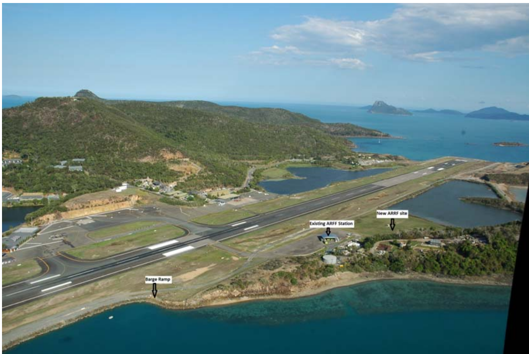
Figure 3: Proposed site location of the new ARFF facility in comparison to the current facility.
