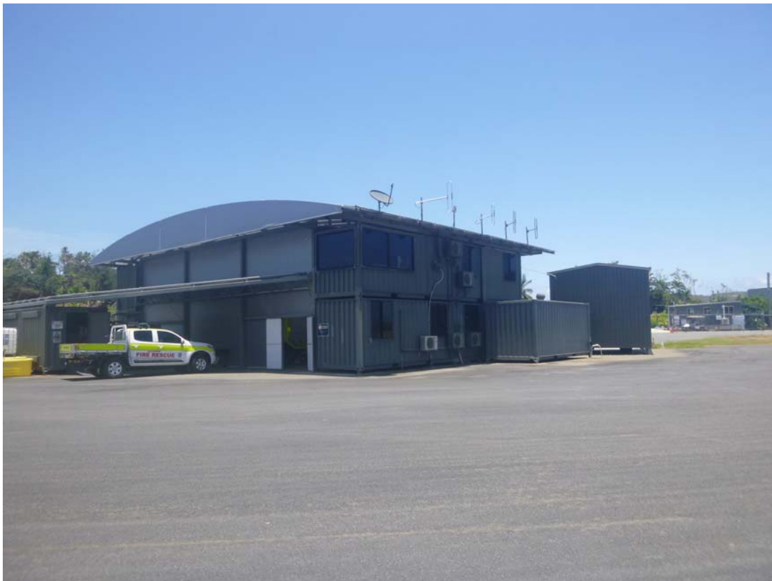
Figure 2 – Existing temporary ARFF facility at Hamilton Island
