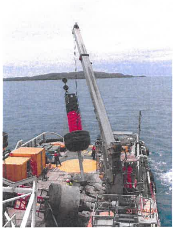
Difficult, specialised work
