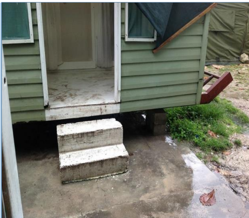
Figure 5: Shower Facilities at Manus Island.
