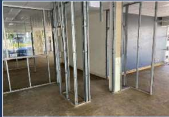
Refurbishment or construction of existing Electorate Offices.
