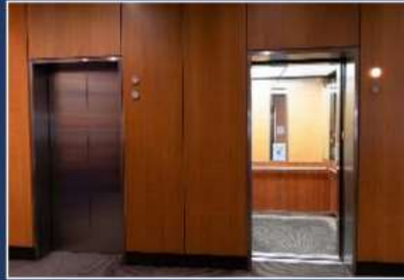
Passenger & Service Lifts Project
