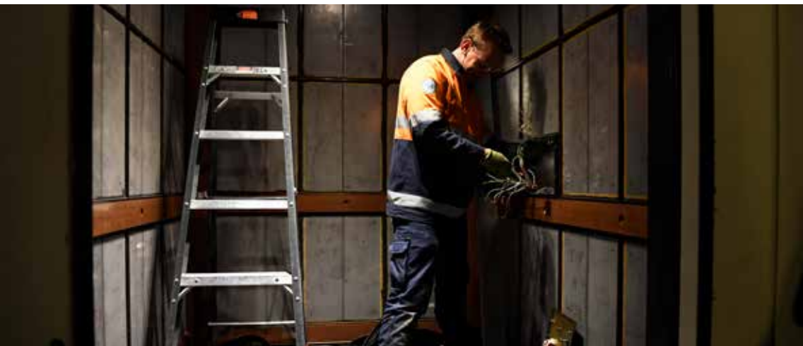
Lift contractor upgrading one of 42 lifts at Parliament House [Auspic]
