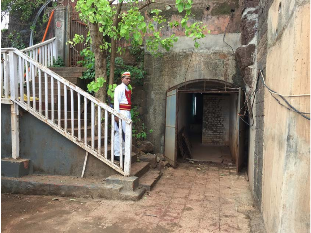
The entrance to the bunker that had been hidden behind vegetation for over a century
