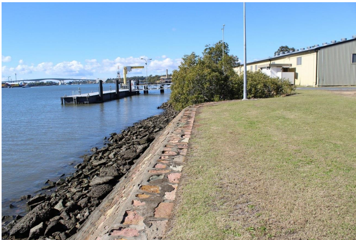
Figure 35: Section of sea wall that will have 2 water pipes inserted to assist storm water drainage from the site. (GML 2017)
