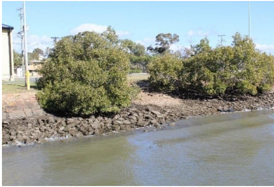
Figure 10: Current break in the sea wall, viewed from the pontoon. (GML 2017)
