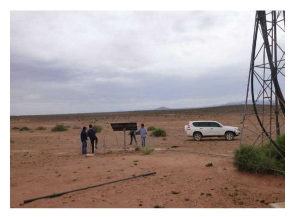
Well 6534-360 (East Yallala Bore) replacing 6534-25, solar pump relaces windmill for stock water.
