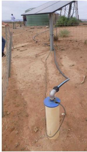
Well 6534-360 pump, power and tank set up.
