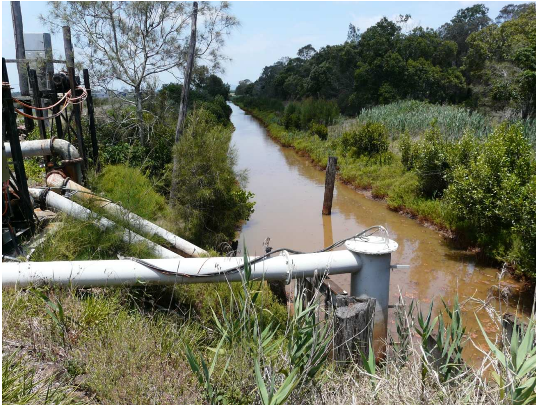
Figure 5. Northern end of western effluent channel at farm 3, looking south. The canal was blocked here at the northern end around 11 am on Monday 5 th and is beginning to fill up at quite a rate. This will need to be decontaminated before being allowed to empty again into the river.
