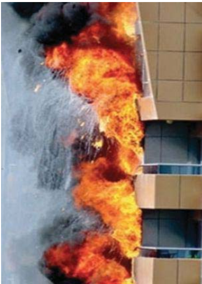
Photo – care of Fire Middle East
