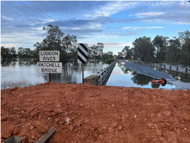
Flood water rising over Patchell Bridge west of Kerang. Photo taken by Belinda Batchelor.
