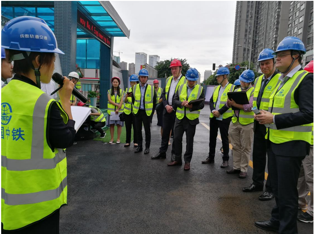
The delegation visiting a construction site for the Chengdu metro.
