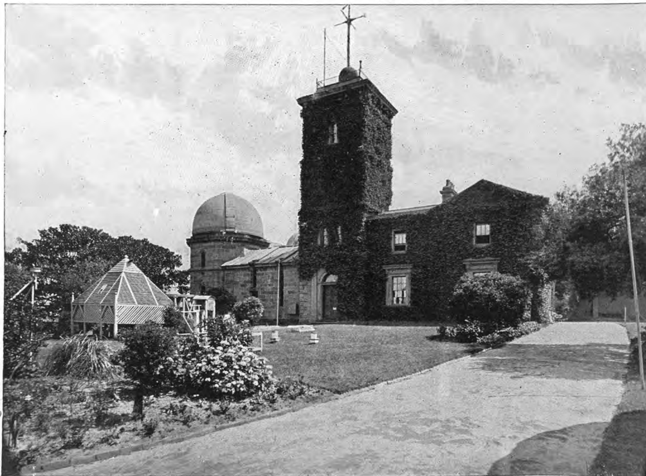
The Observatory. On Flagstaff Hill, the highest point in Sydney, commanding a fine view of the City and Harbour. 10 minutes' walk from G.P.O.
