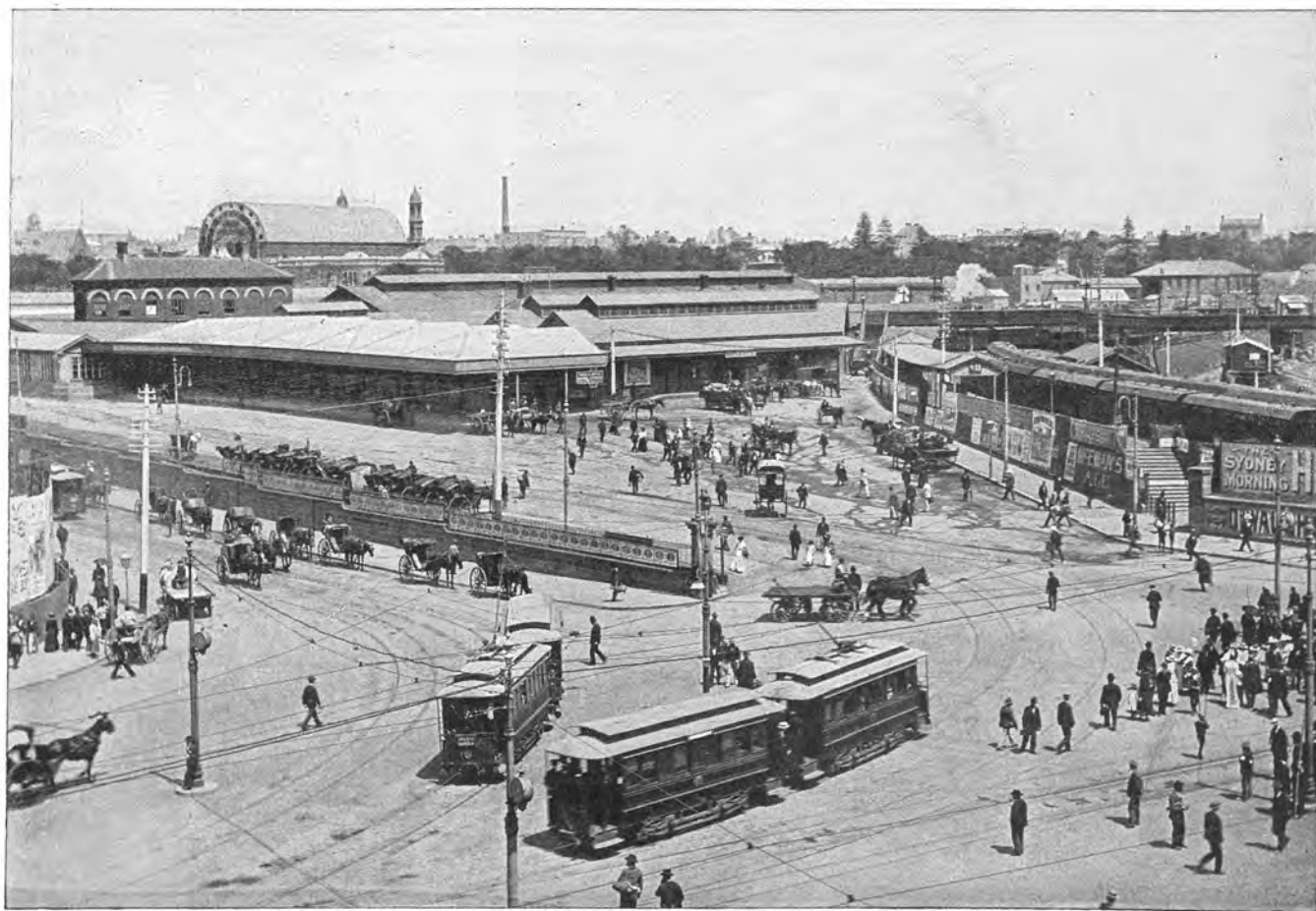
Railway Station. Old Exhibition Building and Prince Alfred Park in the background. A splendid service of Electric Trams connects with Circular Quay.
