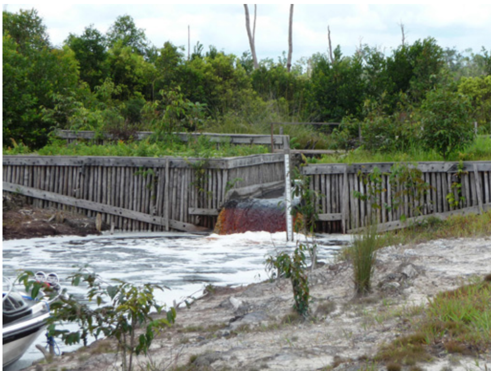
A canal constructed in Sebangau National Park to restore natural peatland hydrology
