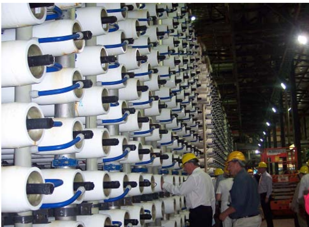
Figure 5 Inspection of Ashkelon desalination plant
